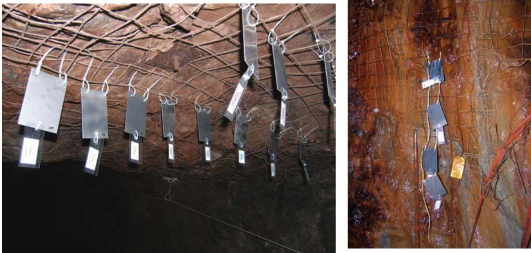
Figure 3. a) Corrosion coupons attached from the mine screen at the back of a drift; b) Coupons installed in flowing water along a drift wall
