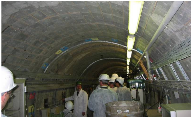
Figure 2. HADES Underground Research Facility, Mol, Belgium (R. Read).
